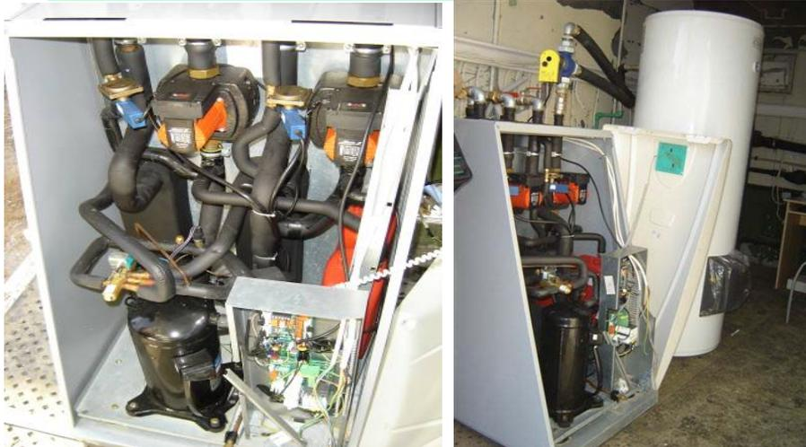
**Fig. 7:** Groundhit heat pump prototype for warm groundwater at the Neo Ryssio demonstration site.
